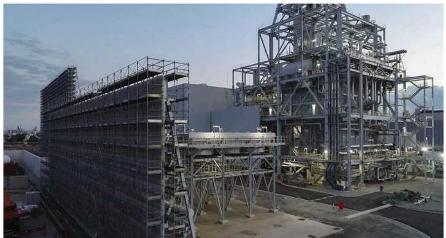
5. Power plants are loud and that can be a problem when neighbors are close to the facility. To reduce noise pollution, MHPS installed soundproof barriers, such as the wall being constructed on the left of this image. Courtesy: MHPS
