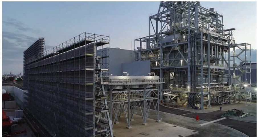
5. Power plants are loud and that can be a problem when neighbors are close to the facility. To reduce noise pollution, MHPS installed soundproof barriers, such as the wall being constructed on the left of this image. Courtesy: MHPS
