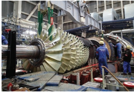
2. MHPS’s J-series gas turbines are an integration of the proven G-series design. The M501JAC adopted air cooling for combustors instead of steam cooling, which produces a high level of operability including a shorter start-up time than the M501J. The gas turbine rotor is shown here being lowered into the casing. Courtesy: MHPS
