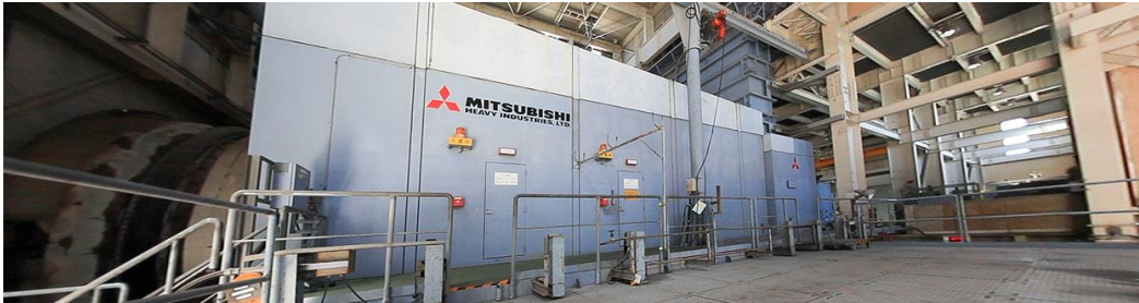
Figure 5. Validation Plant Standard Enclosure
